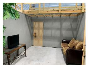
Breaching doors designed for forcible entry using battering rams or ballistics feature replaceable lockset panels. The facility also includes a window for sniper training. Accessed from stairs on the side of the structure, the overhead walkway gives trainers a clear view of the exercise and other rooms below.
