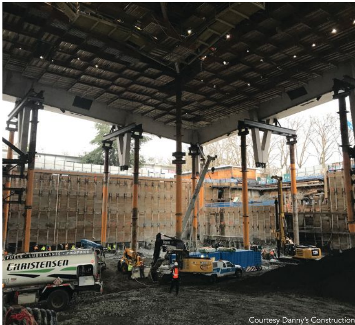
above and left: Temporary roof shoring and excavation. below: W36 beams supporting existing Y-columns.
