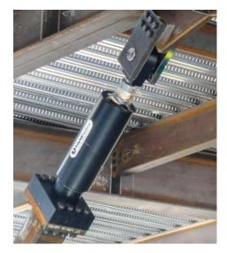
Protect new or existing structures against earthquakes simply and inexpensively. Taylor Devices' Fluid Viscous Dampers provide complete protection for buildings, bridges, towers, elevated freeways - virtually any structure that is subject to earthquake damage.
