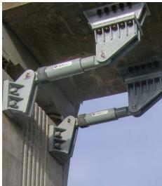
In the 1990s, Taylor Devices began using snubbers, originally developed during the 1960's for protection of large steam pipes in nuclear power plants, as locking devices to limit the relative motion of highway bridge sections under various types of transient motion - usually seismic in origin. When used on civil engineering structures, the product is usually called a lock-up device (LUD) or shock transmission unit (STU).
