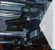
This photograph shows a 7,600 lb TMD designed and manufactured by Taylor Devices used to mitigate lateral movements on a long pedestrian bridge. The mass is suspended by steel cables, tuned to the lateral frequency of the bridge, and is controlled by fluid dampers. One of these dampers is shown in the foreground with heat dissipating fins on its outside diameter.
