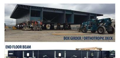
Erection engineering and sequencing for the 2,440-ton main span, comprised of triple steel box girders with integrated orthotropic steel deck, and permanent lift span towers and counterweight.
