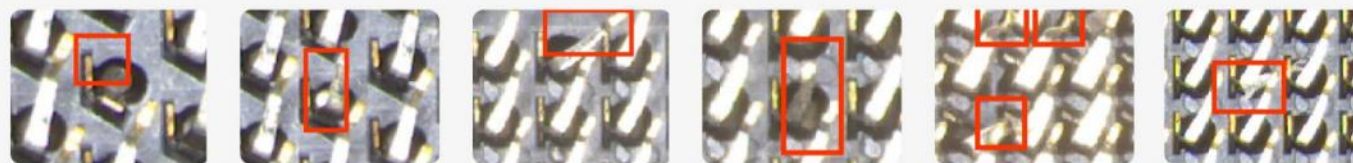
Missing Broken Shift Sank Deformation Foreign matter
