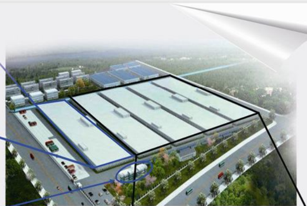
待建设的其他四期厂房 Other 4 phases are under construction planning
